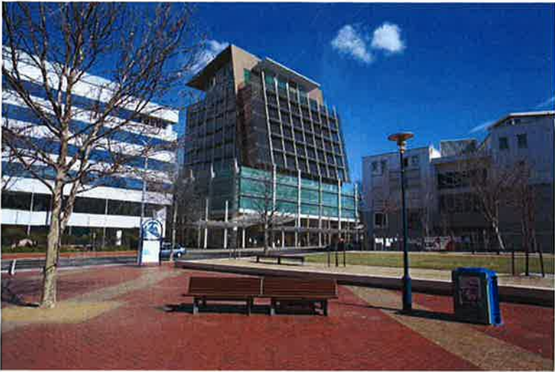
VIEW FROM NORTH EAST
